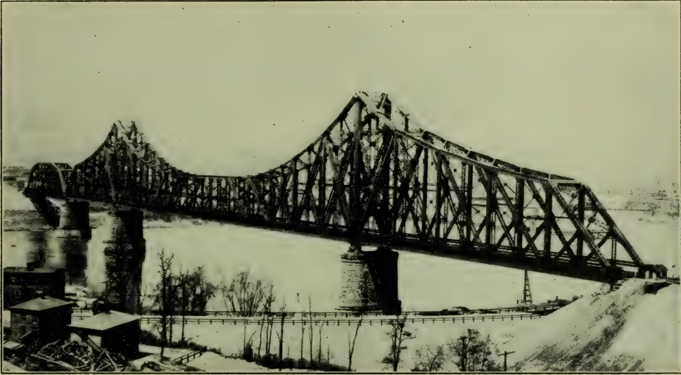
FIG. 6A.—Beaver Cantilever Bridge, across the Ohio River (769 Feet Channel Span)
